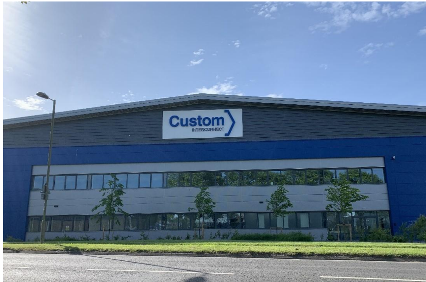
BP2 UK's largest Semiconductor Packaging facility (OSAT) + Volume PCBA manufacture 64,000sq ft
